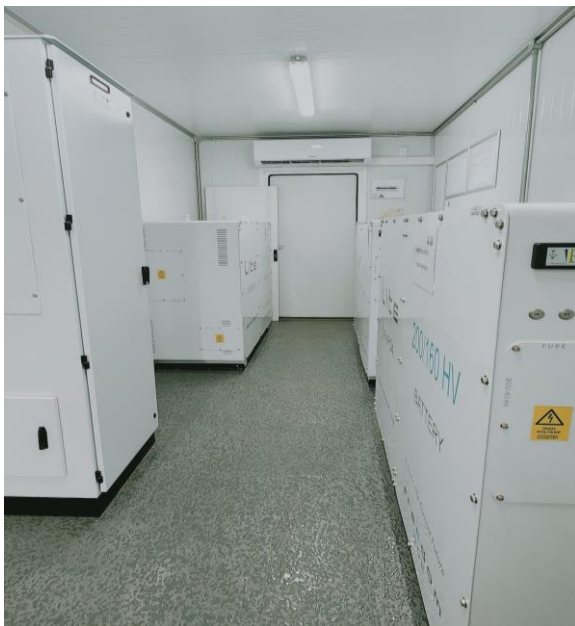
Lenasia City power offices (270kwp, 600kwh battery in container)
